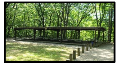
Rotary Pavilion 34' x 60' structure
